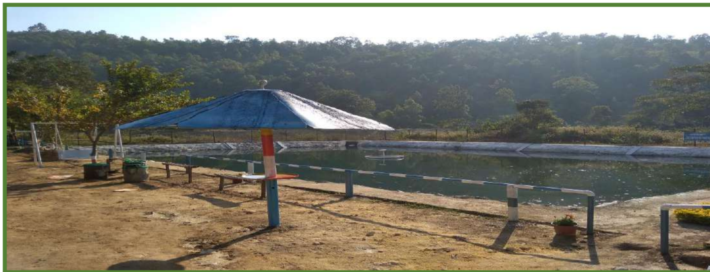
SETTLING POND, NO – 3
