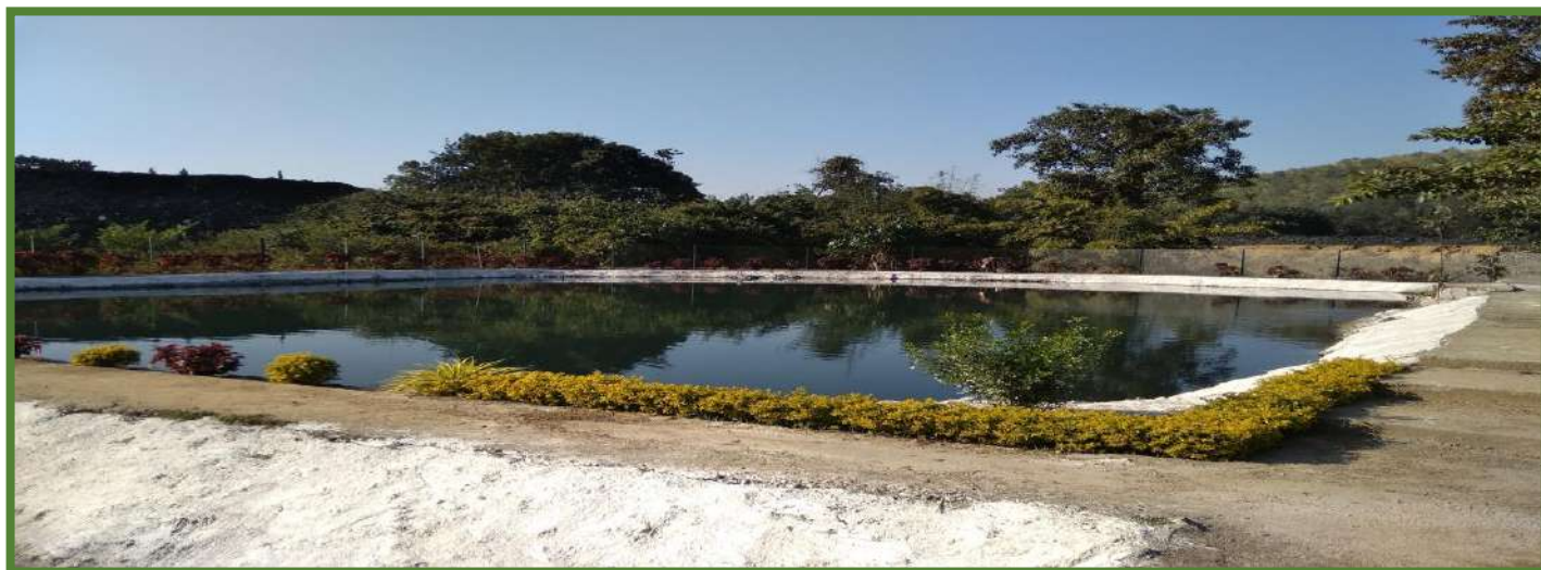
SETTLING POND, NO – 2
